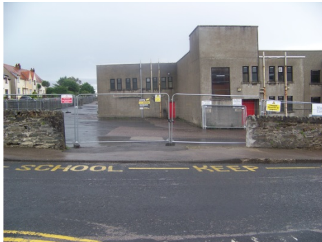
6a Existing school buildings to be demolished
