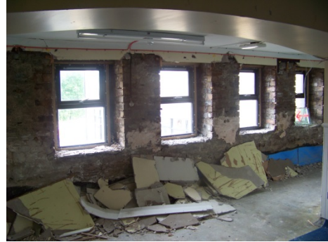
5b Pre- Demolition - "soft strip" of existing buildings
