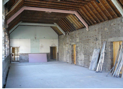
4 Existing 1881 school building "retained shell"
