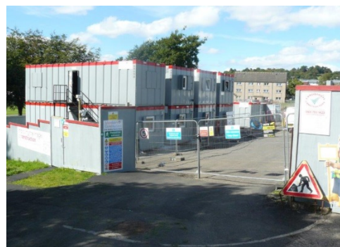
2 Site offices to the rear of 1881 building
