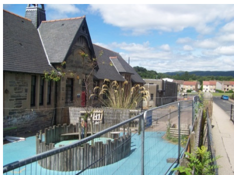
1 Existing 1881 school building to be retained.
