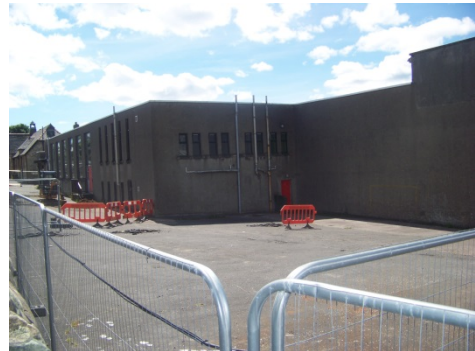
6b Existing school buildings to be demolished
